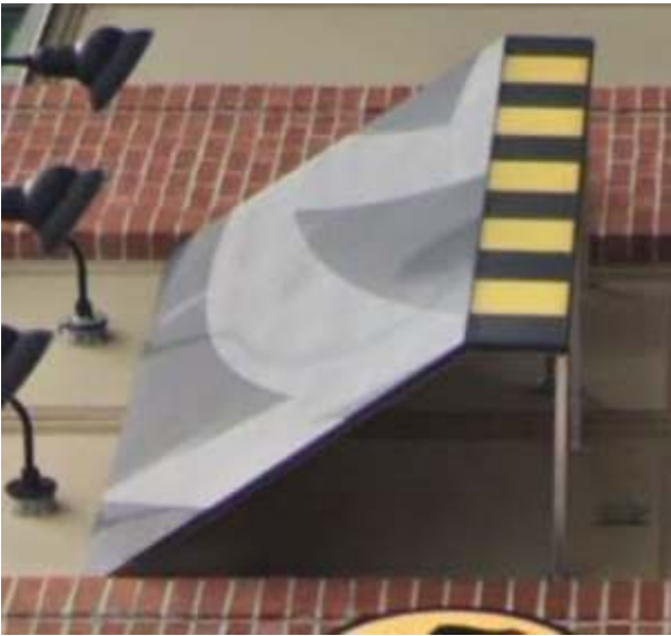
EXISTING AWNINGS ARE OPEN ENDED
