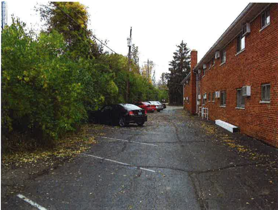
View from the southwest property corner facing north along the west property line and existing building #4
