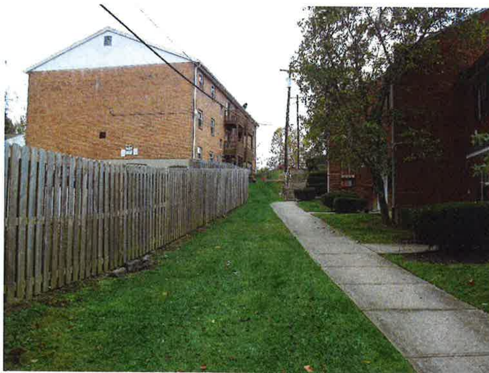
View from the southeast property corner facing southwest along the south property line and building #6
