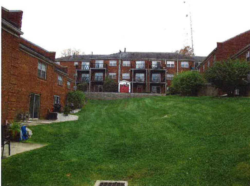
View from the east property line facing west towards building #6
