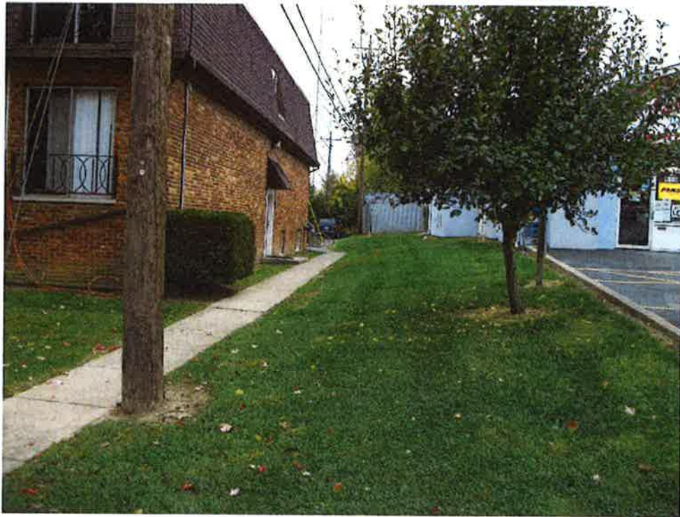
View from the northwest property corner facing south along the west property line of existing building #1
