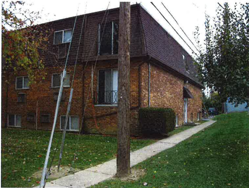
View from the northwest property corner facing southeast towards existing building #1
