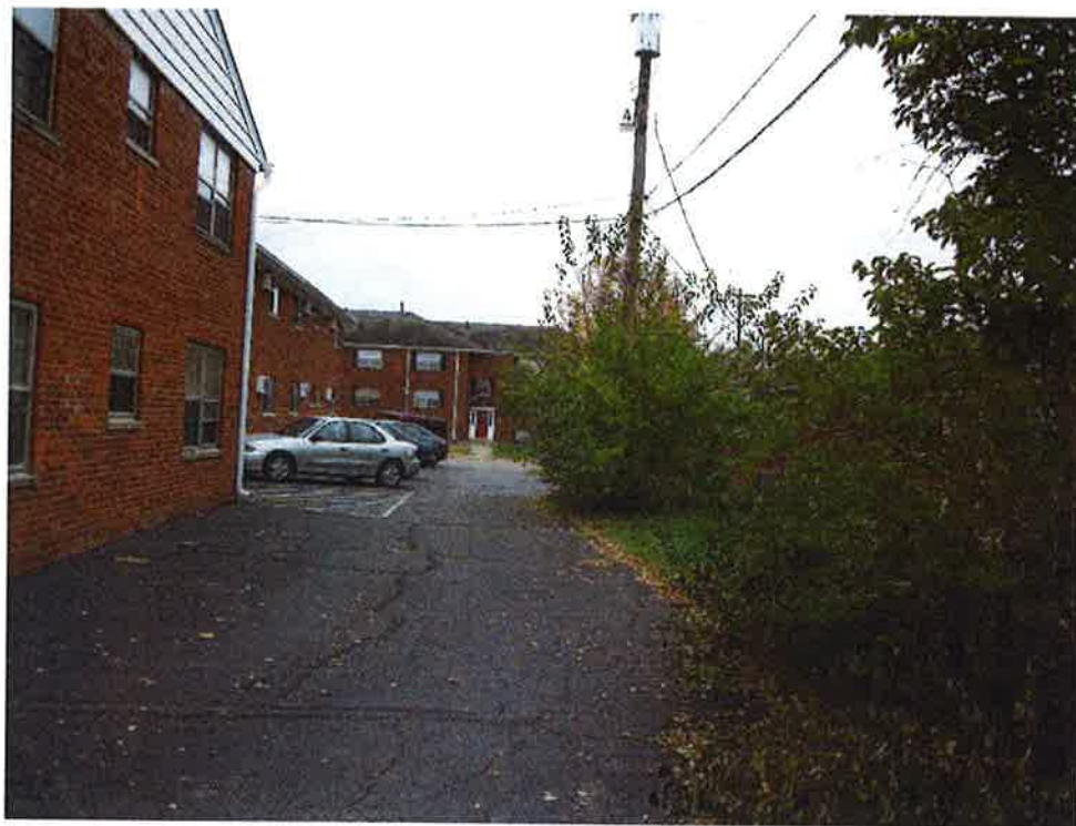
View from the southwest property corner facing northeast along the south property line along existing building #4
