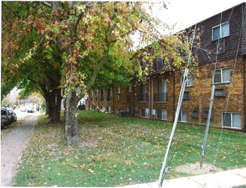
View from the northwest property corner facing east along the walk of Chestnut St. and existing building #1
