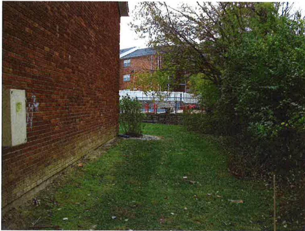
View from the southeast property corner facing north along the east property line and building #6
