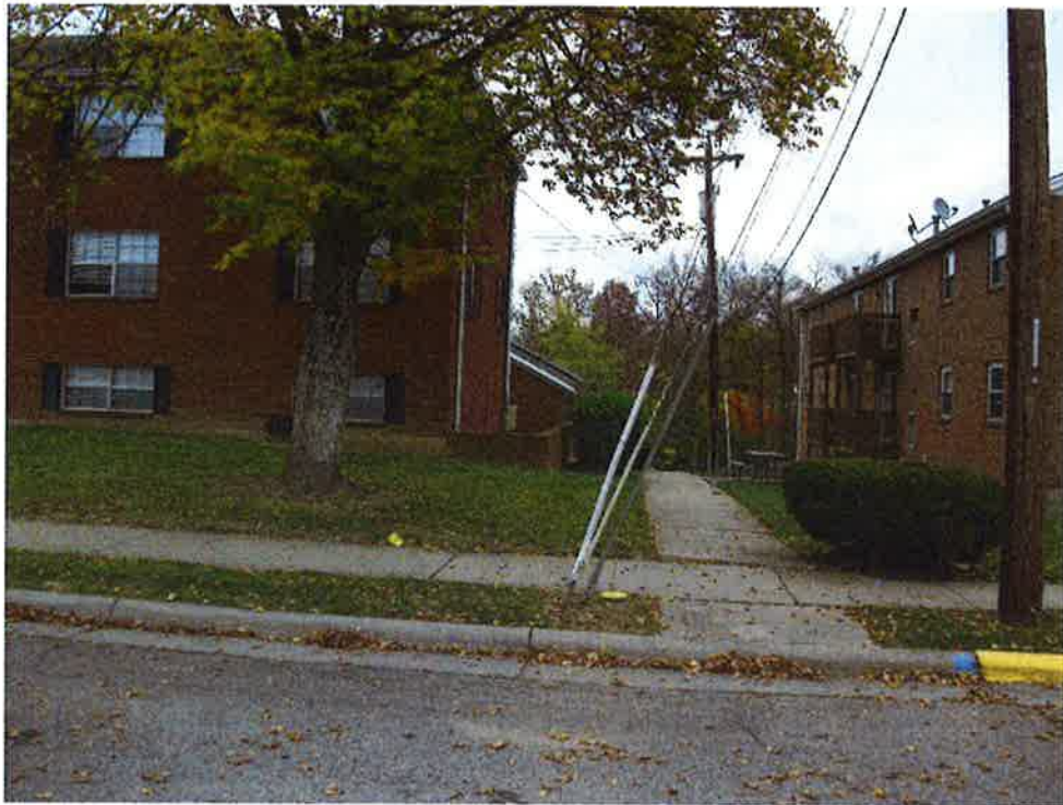
View from the center of Arrowhead Dr. at the south property line facing northeast along existing building #6
