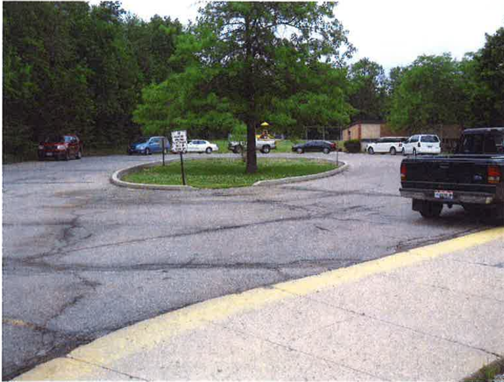
View of the entrance loop.
