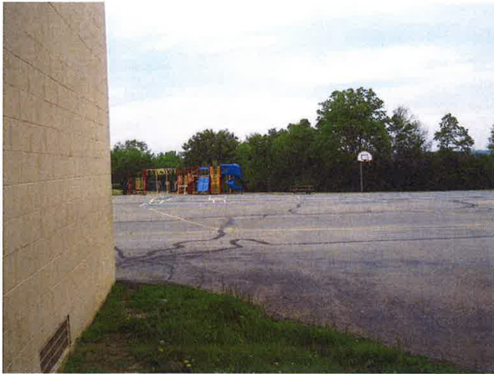
View from the north side of building facing north.
