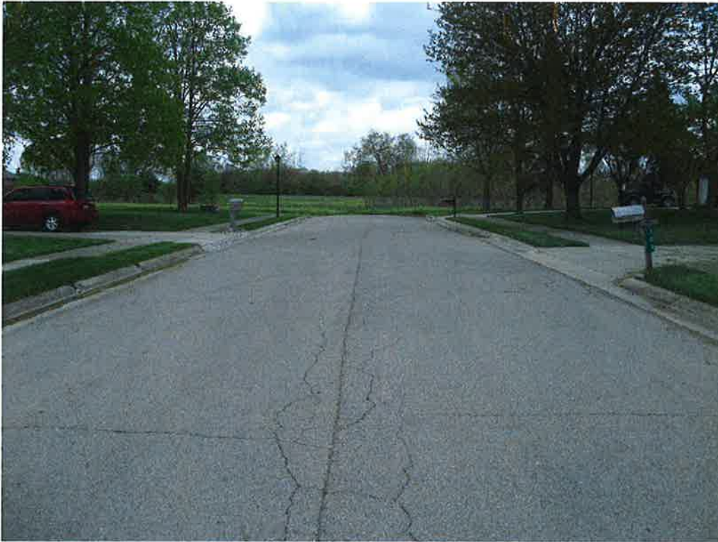
View from the center of Olde Farm Road looking North.
