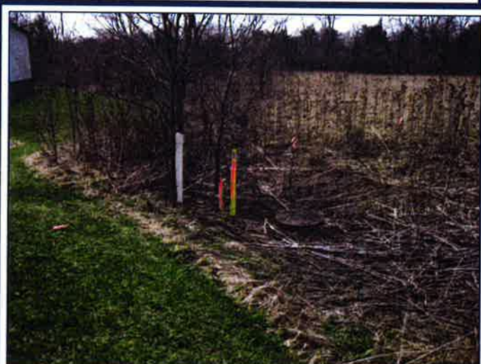
8 - Sanitary Sewer MH Near South Corner
