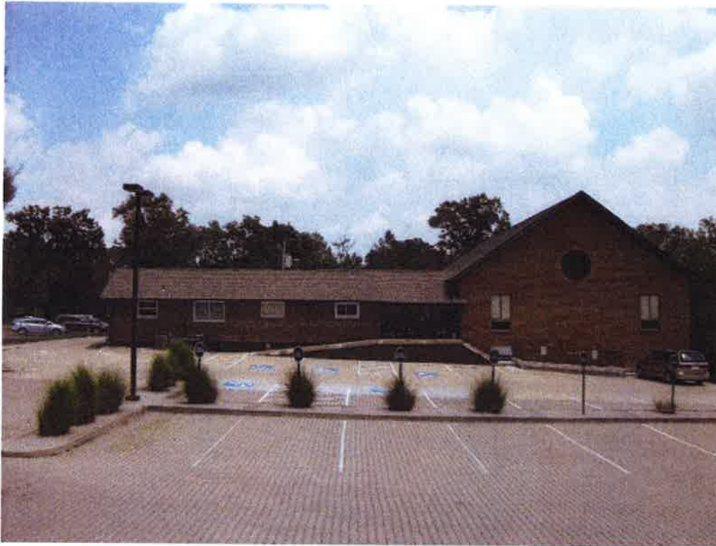
13) View from the west property line facing east.
