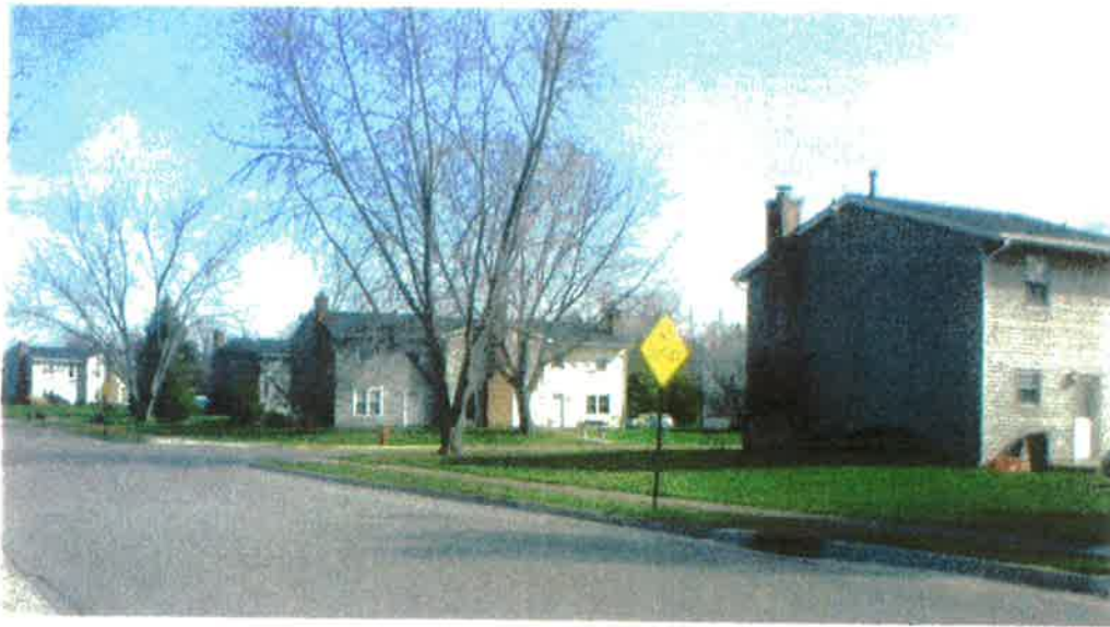
Existing R-3 Development across Jaqueline Drive
