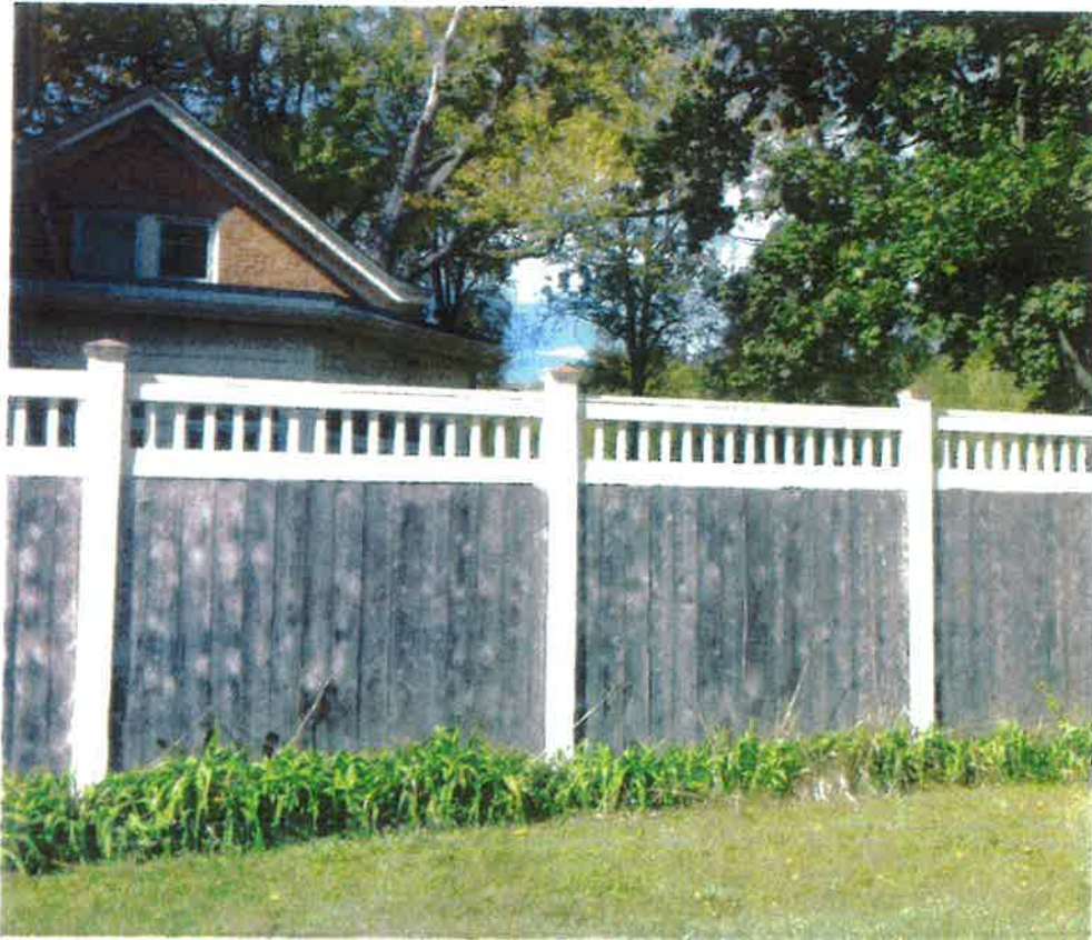
Existing Privacy Fence along Jacqueline Drive
