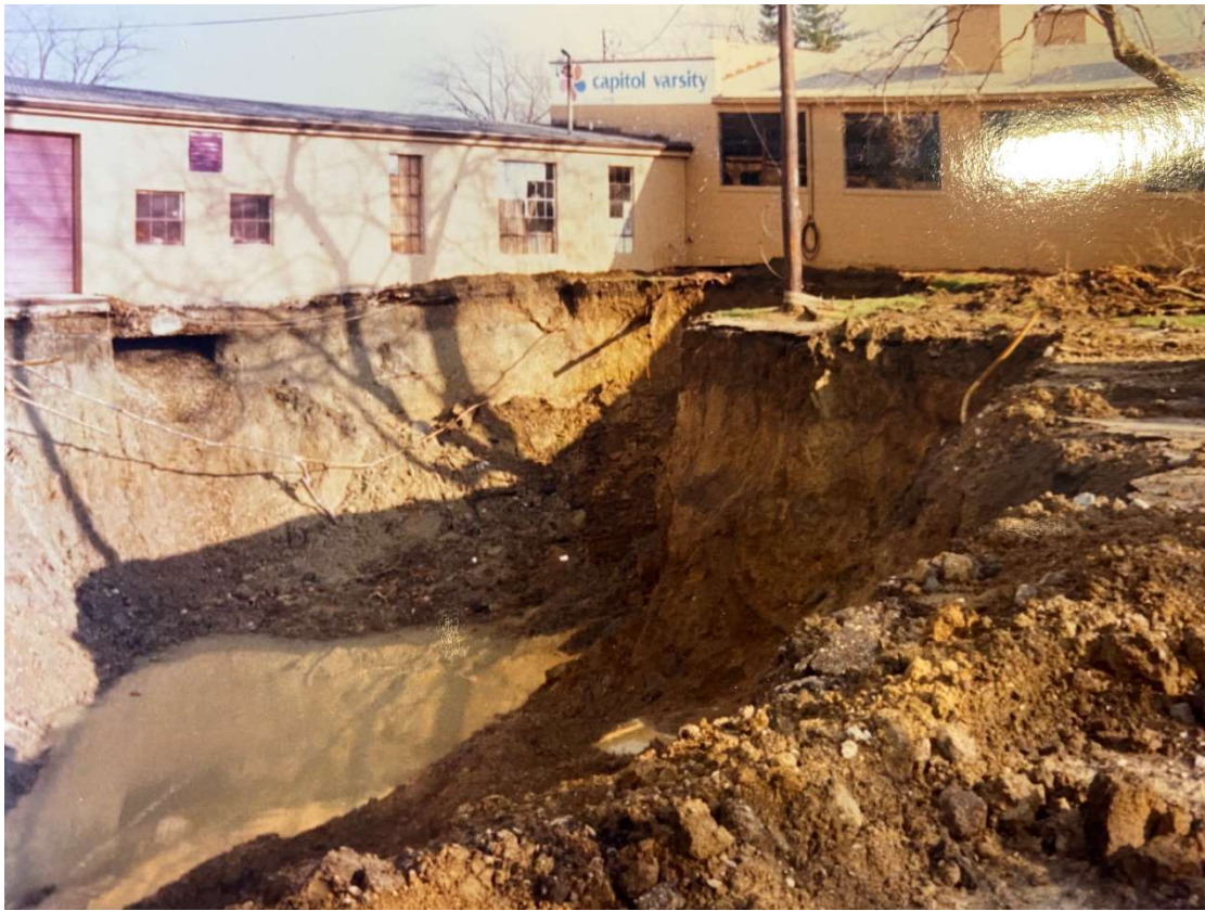
Excavation of parking lot, west face of original office building.
