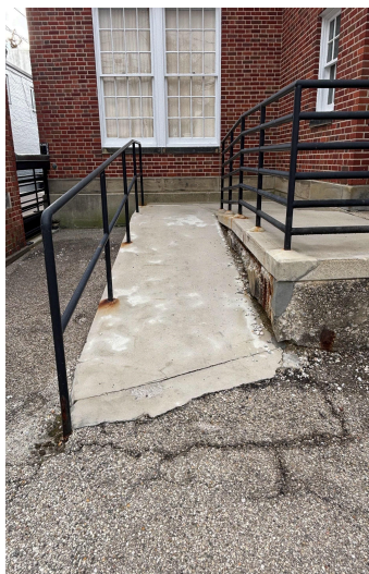
Uneven ramp that is covered in rocks and pebbles, making a difficult transition from the road. Additionally, the ramp is only wide enough for one person at a time, meaning people would have to walk in a line rather than next to each other.
