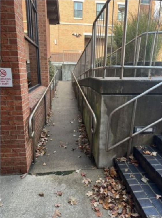
Image 1.3 *Image shows the ramp, at the entrance with the attached parking lot, with a narrow ramp.
