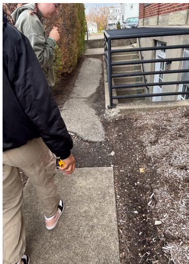
Uneven sidewalk on the side of the building closest to the curb cut. This makes it difficult or impossible for disabled people to access the accessible entrance from this side.
