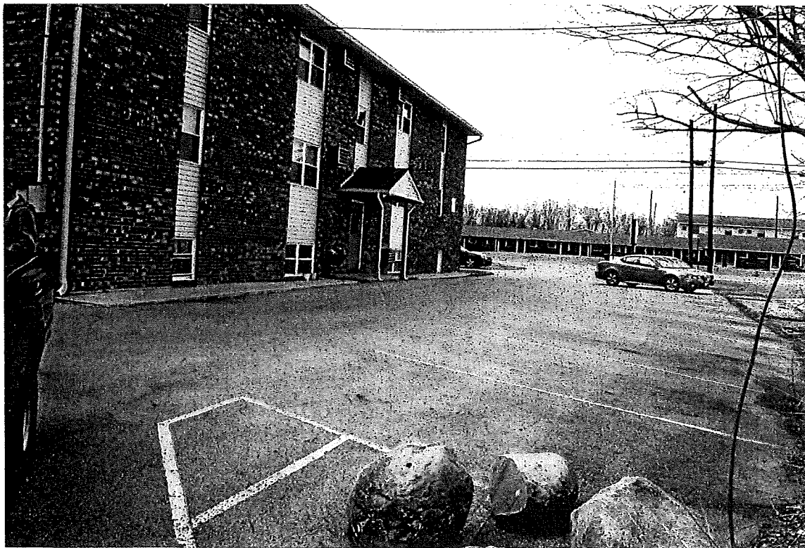
North side parking from northeast (front)
