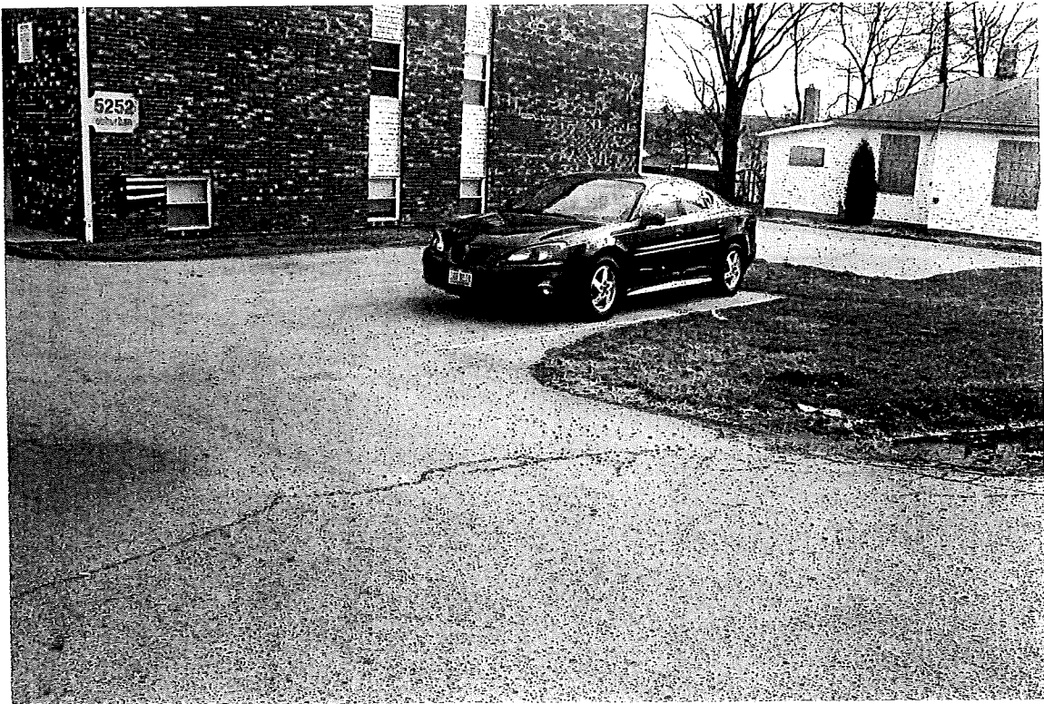
Front parking from northwest
