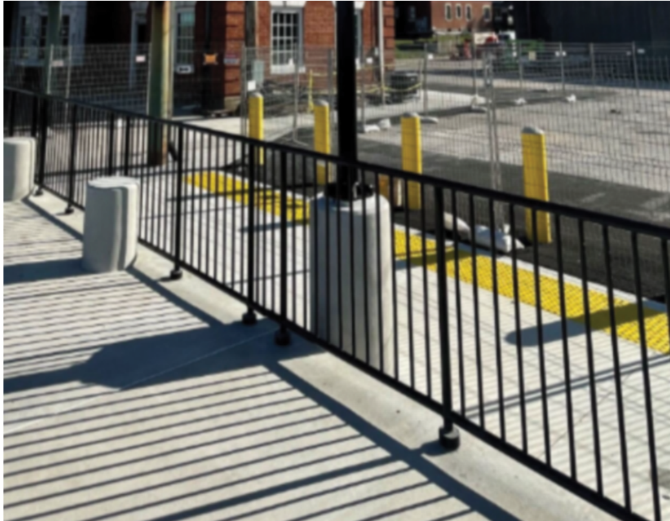
Railing - 4' Height to match Maysville/Connersville Platforms
