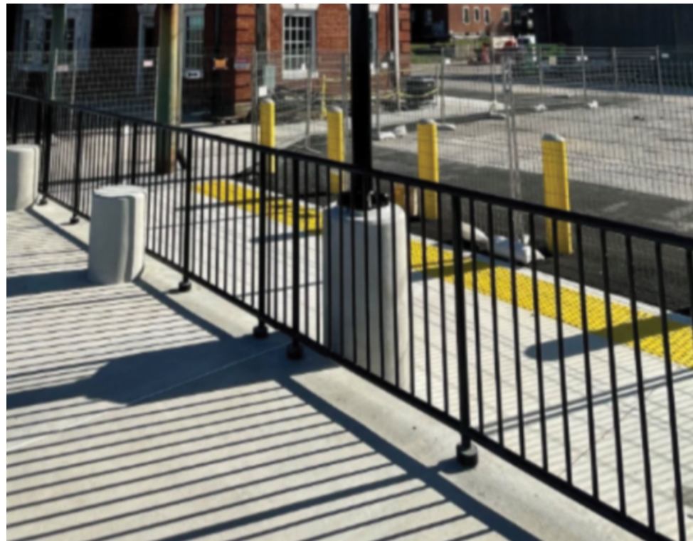
Railing - 3'-6" Height to match Maysville/Connersville Platforms
