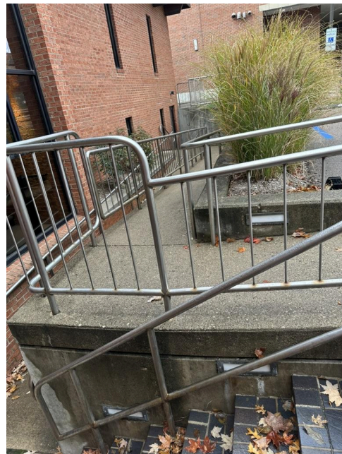
Image 1.4 *Image shows the ramp, at the entrance with the attached parking lot, with a ramp that has several narrow turns.
