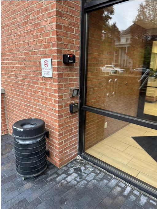
Image 1.1 *Image shows the automatic door opener on the opposite side of the entrance to which the door is located.
