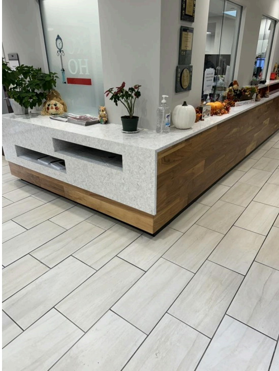
Image 2.4 *Image shows that there is no overhang on the countertop ledge.
