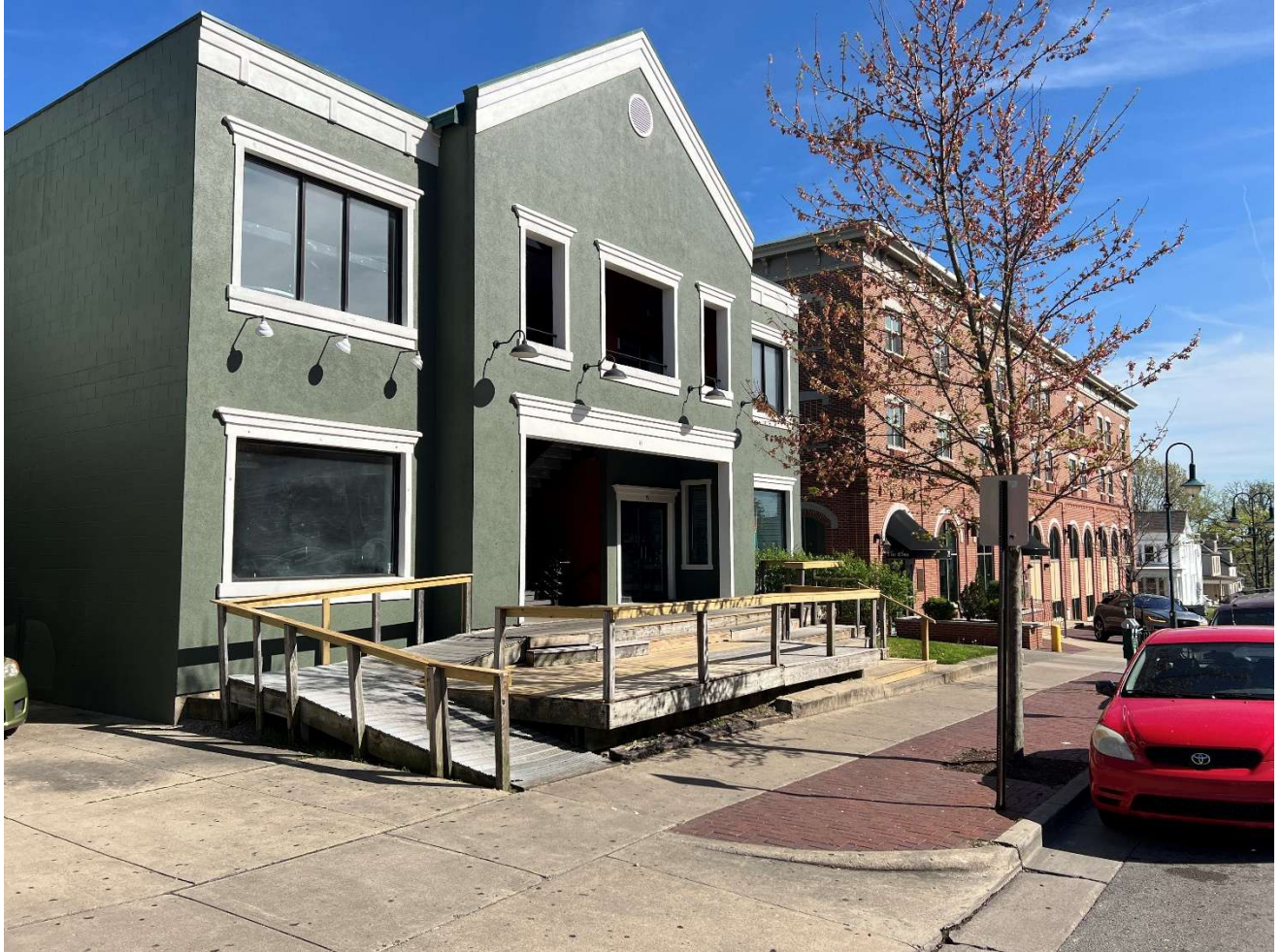
Existing Building along S Main Street
