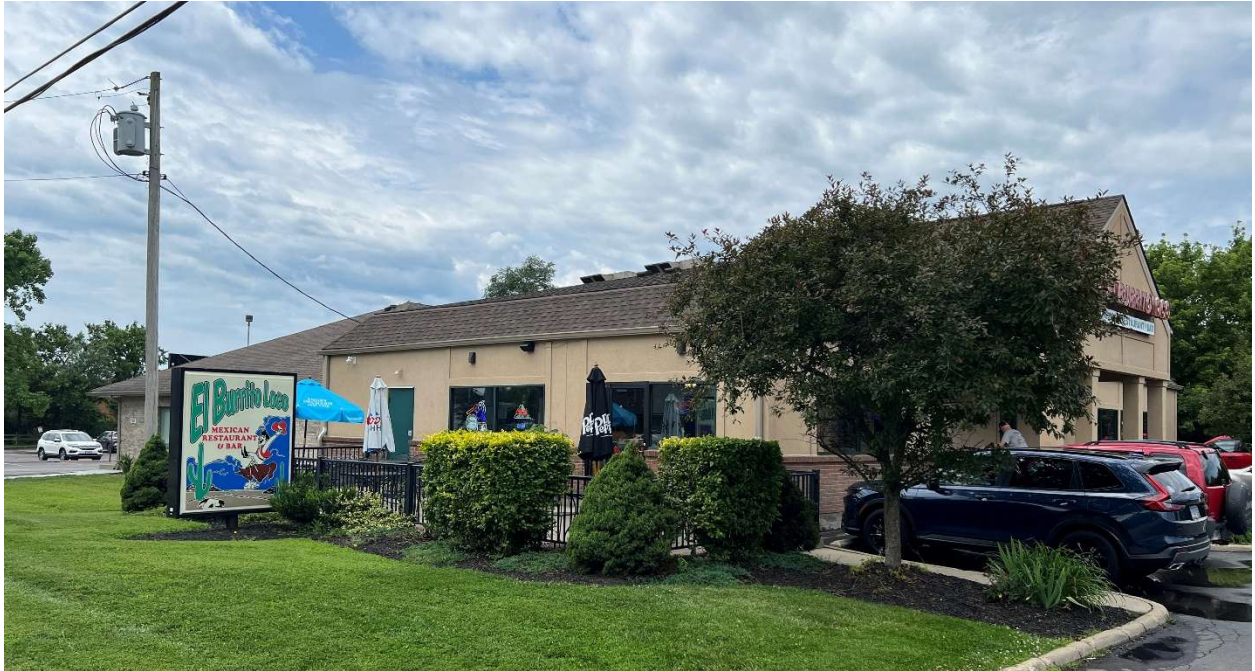
Existing Building along S Locust Street
