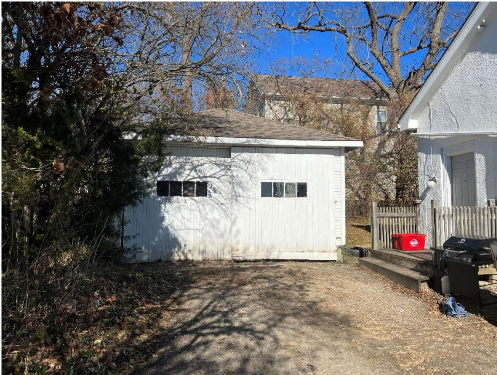
Existing Garage to be re-used
