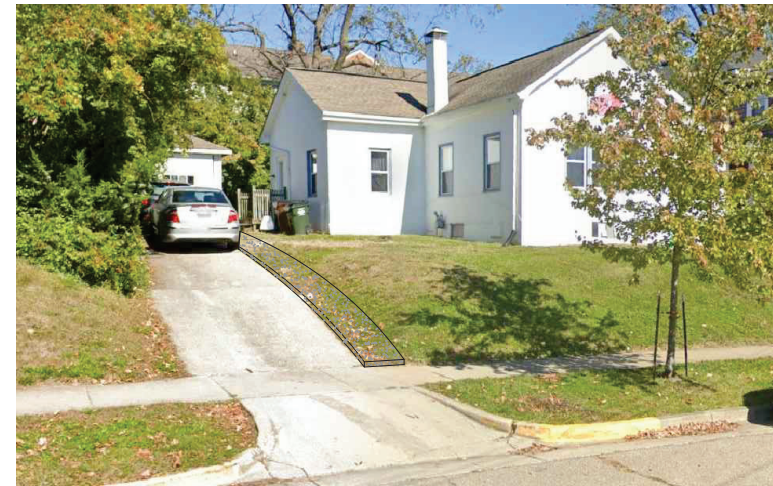
SITE PHOTO \frac{1}{4}" = 1'-0" SHOWING NEW SIDEWALK
